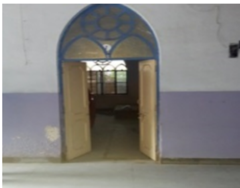
Building Front View
