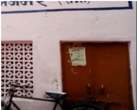
Building Front View
