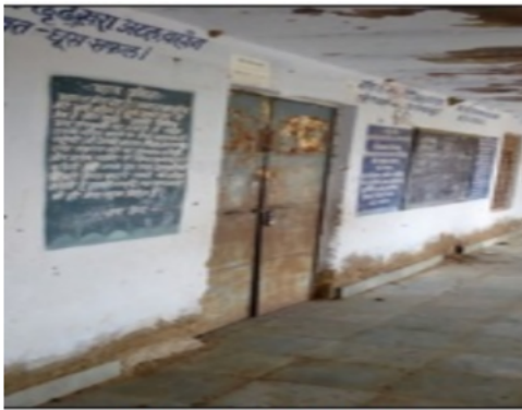
Buildina Front View
