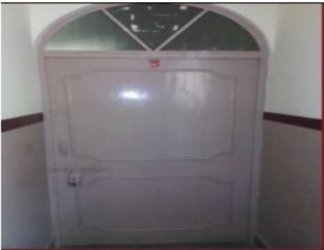
Building Front View
