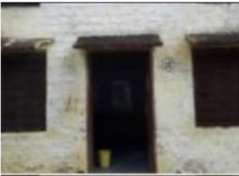
Building Front View
