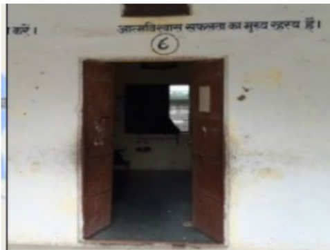
Building Front View
