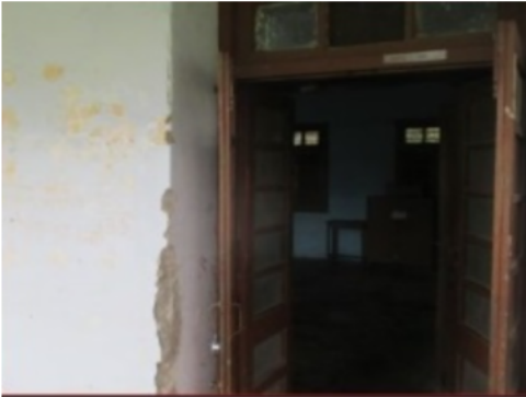
Building Front View
