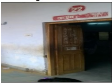
Building Front View
