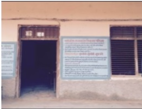
Building Front View
