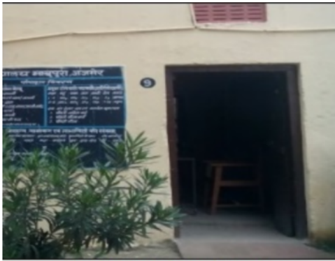
Building Front View
