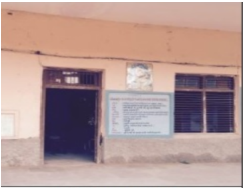
Building Front View
