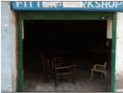
Building Front View
