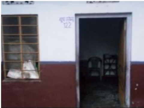
Building Front View
