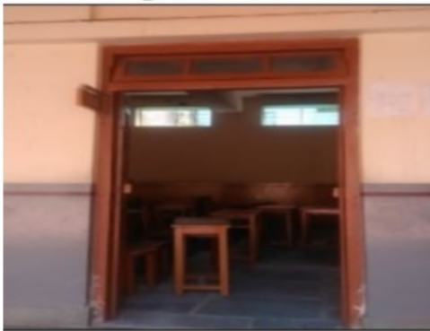
Building Front View
