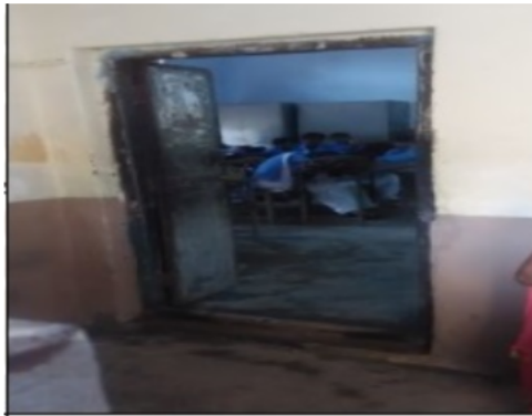
Building Front View
