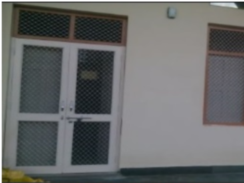
Building Front View
