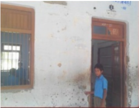
Building Front View
