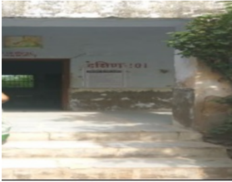
Building Front View
