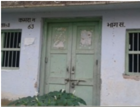
Building Front View
