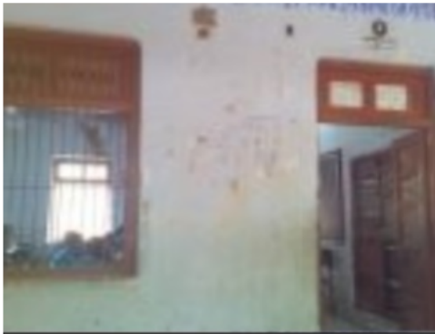
Building Front View
