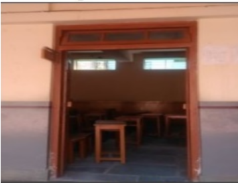
Building Front View
