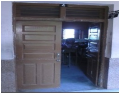
Building Front View
