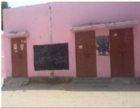
Building Front View
