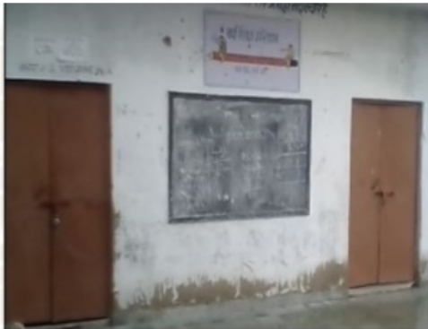
Building Front View
