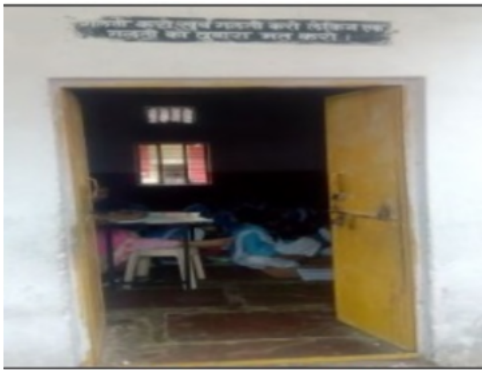
Building Front View
