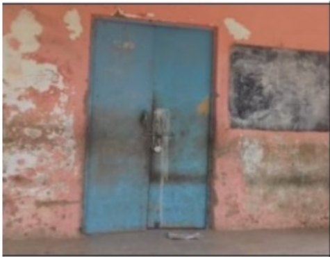
Building Front View
