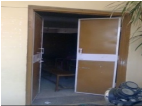
Building Front View
