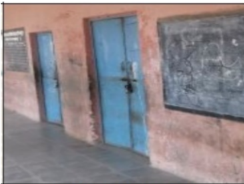
Building Front View
