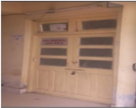
Building Front View
