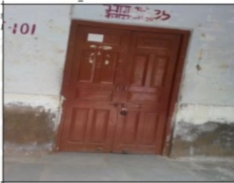
Building Front View
