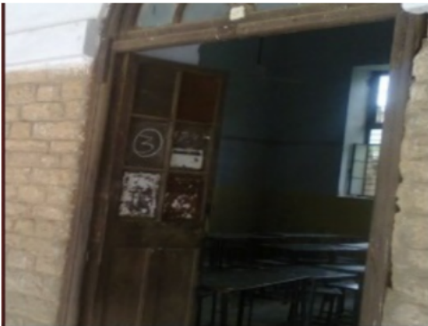
Building Front View
