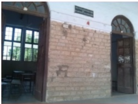
Building Front View
