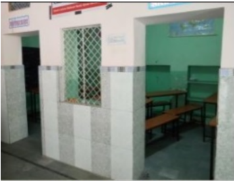
Building Front View
