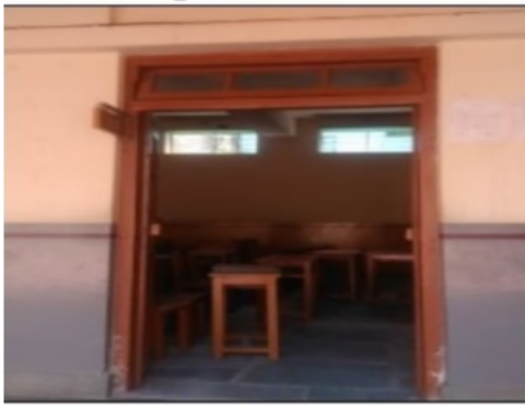
Building Front View
