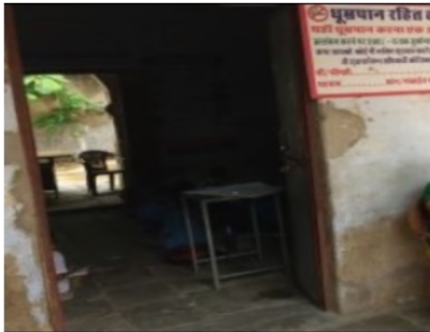
Building Front View
