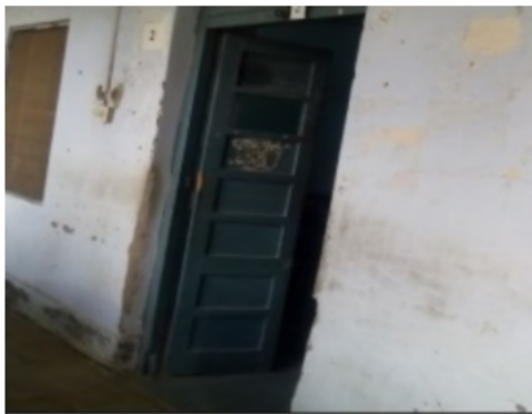
Building Front View
