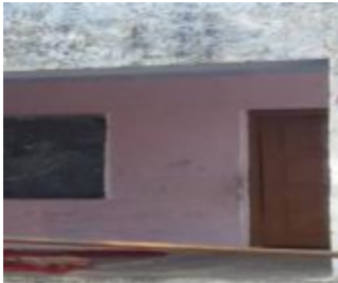
Polling Station Building Front View
