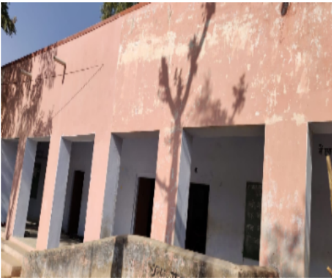
Polling Station Building Front View
