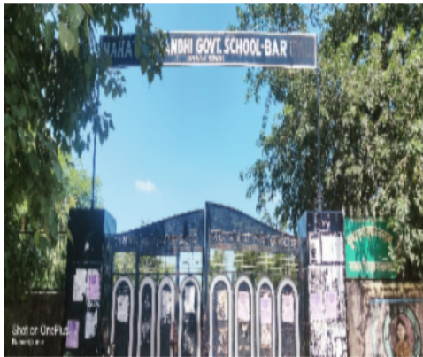
Polling Station Building Front View
