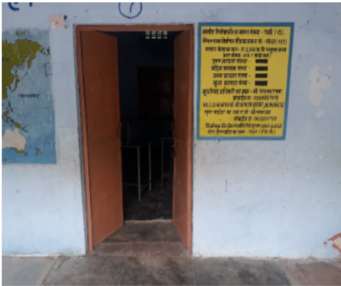
Polling Station Front View
