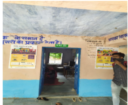
Polling Station Front View
