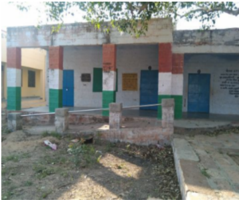
Polling Station Front View
