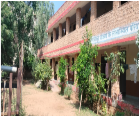
Polling Station Front View
