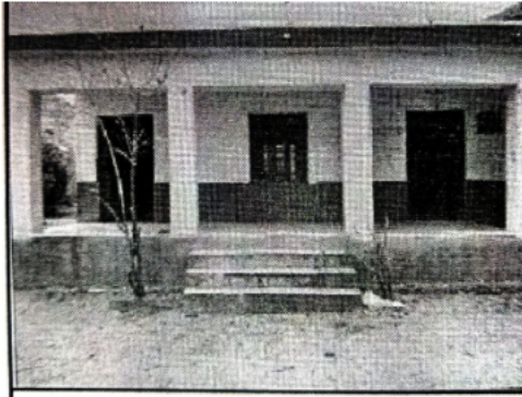
Building Front View
