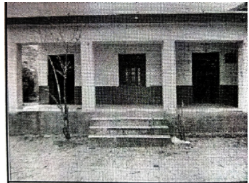
Building Front View
