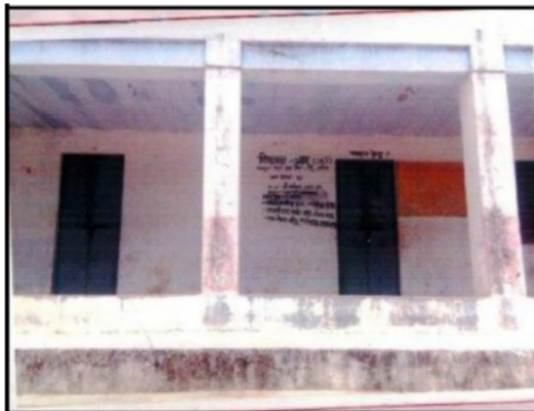
Building Front View
