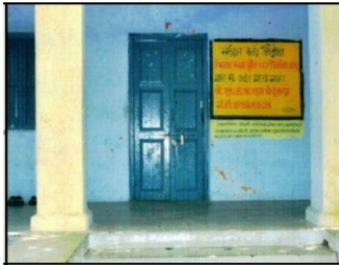
Building Front View
