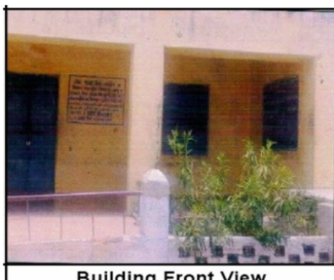
Building Front View
