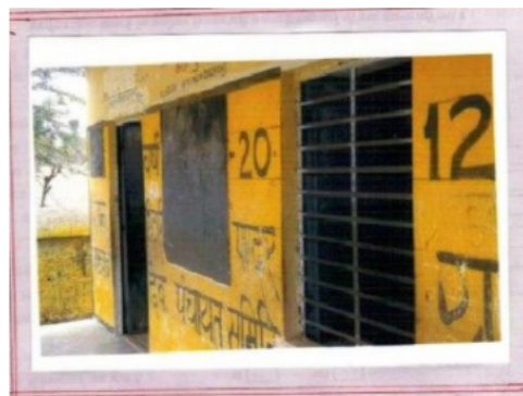
Building Front View
