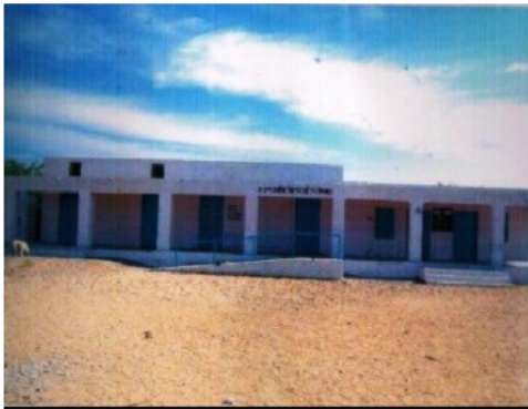
Building Front View
