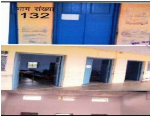
Building Front View
