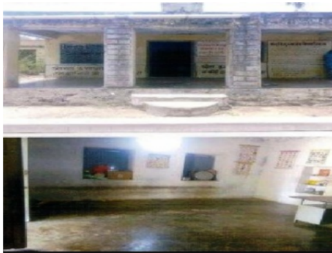
Building Front View
